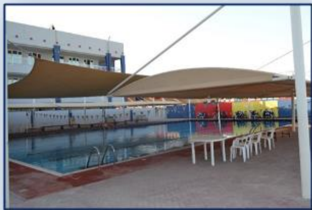
New shading for the big swimming pool has been installed
